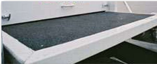
Beverage truck deck after FIRM GRIP has been applied.
