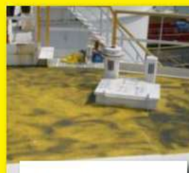
Top of a petroleum storage tank
