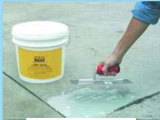
SURE PATCH being applied to a warehouse floor
