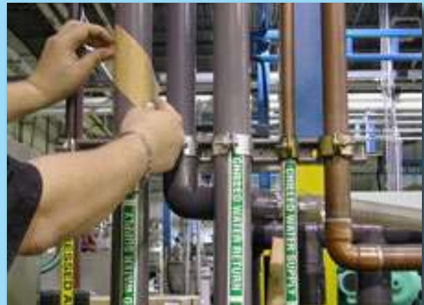
EASY PATCH being applied in a mechanical room at a manufacturing plant
