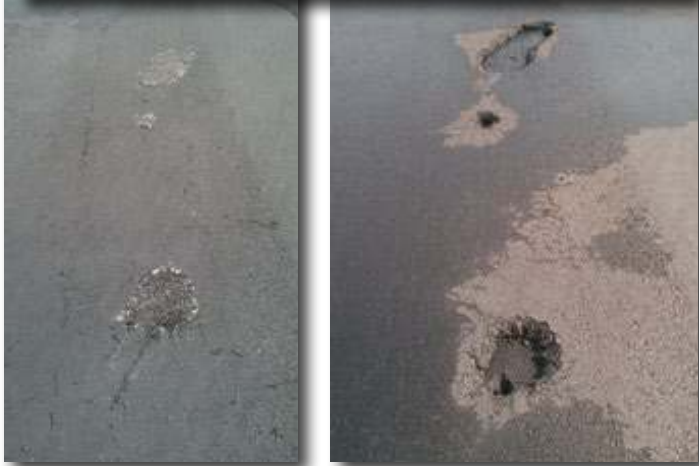
TRUE BOND PATCH applied to an airport runway
